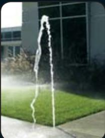
At 40 psi, the standard pressure fixed spray with a missing nozzle wastes water at a rate of 40 GPM.
